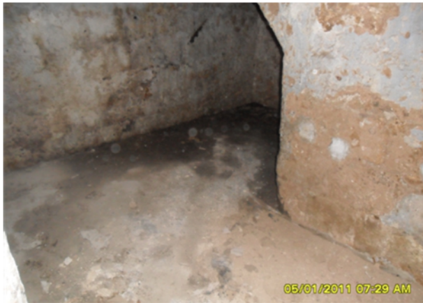
Before Concrete slabs Demolition Block A- Ground Floor, Room 129
