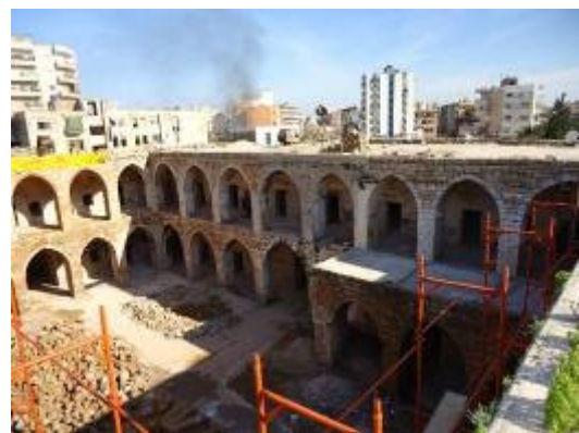
Khan A: north west interior elevation - Demolition and removal of all concrete harmful interventions
