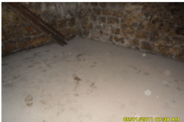
Before Concrete slabs Demolition Block A- Ground Floor, Room 114
