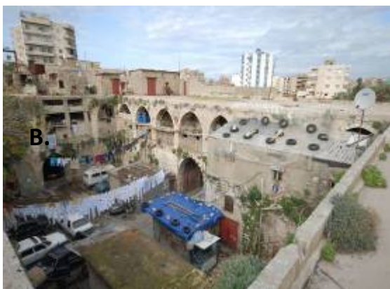
Khan A: south west interior elevation - Demolition and removal of all concrete harmful interventions
