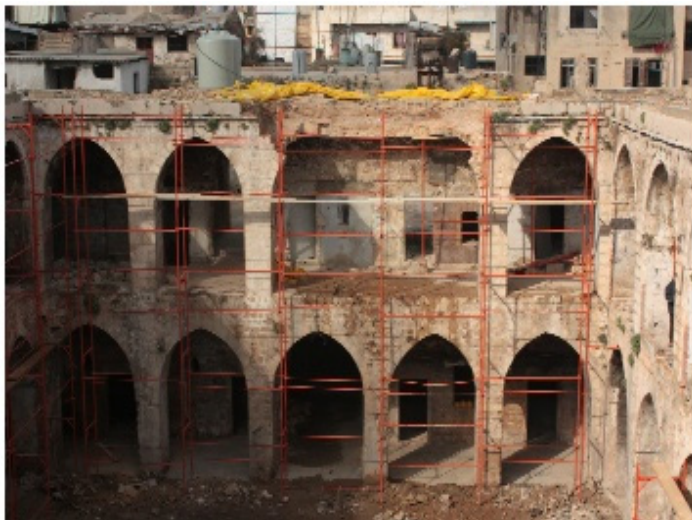
After removing the concrete structure
