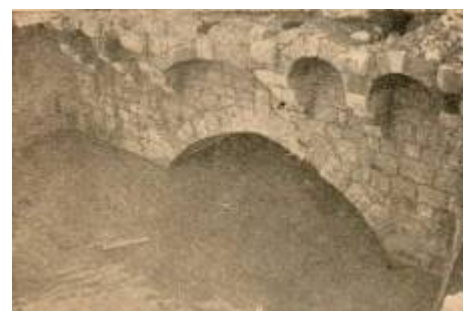
The Lahhamin bridge
