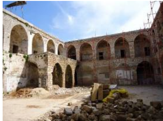
Khan A: north west interior elevation - Demolition and removal of all concrete harmful interventions
