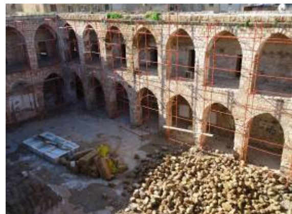
Khan A: north east interior elevation - Demolition and removal of all concrete harmful interventions
